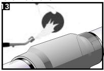
Heat the adhesive side of the CFS with a medium intensity flame until the adhesive serrations disappear (adhesive will melt).
