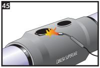
Using a weak medium flame, heat the backside of the CFS until the adhesive oozes from the edge and the thermochromic ink print disappears. **Do not overheat the surface as the foam will gas**.
