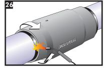
Using broad strokes and a medium flame, begin shrinking one end of the CSC evenly all around. Keep the torch moving to avoid overheating any spots; ensure sufficient heat is applied at the bottom.
