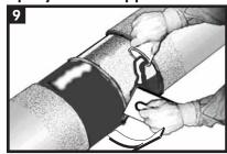
Apply mixed epoxy to a minimum uniform thickness of 4 mils on all exposed bare metal plus 10 mm (0.5") onto the adjacent pipe coating.
