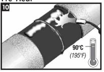
Pre-heat the epoxy and the abraded coating to  $90^{\circ}C + -5^{\circ}$  ( $195^{\circ}F + -10^{\circ}$ ) with the appropriate propane torch. This will substantially cure the epoxy and ensure proper flow and bonding of the sleeve adhesive. Do not use an intense flame on the mainline coating. If a film develops on the mainline coating because of preheat, use a surface abrasion tool to remove it.
