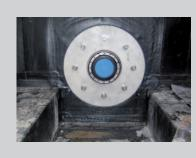
Press-seals and plastic liners are available quickly and inexpensively in all versions, whether 50 mm or 1,500 mm.
