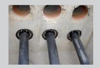
In combination with the P-LINER Basic plastic liners, the press-seals create the perfect combination solution for secure sealing of wall ducts. The profiled rib gasket homogeneously conjoined with the liner provides a reliable seal between the liner and the building, and allows flush placement in the formwork.
