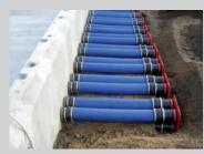
Our special-purpose press seals P-CABLE are the perfect solution for cables in core holes and liners.
