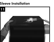
Partially remove the release liner from the sleeve (~15 cm from the edge) and gently heat the adhesive along the underlap with a torch.
