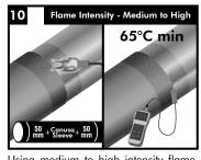
pre-heat and activate the surface to be covered with heat shrink sleeve and **min** 50 mm on each side of the sleeve to a minimum temperature of 65°C. The flame shall be kept perpendicular to the surface of the pipe and casing during pre-heating. Check the temperature around entire circumference of the pipe with a touch probe.
