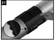
After shrinking, press down on the sleeve to ensure adhesive flow over the entire surface. Special attention should be given along the circumference between 4 and 8 o'clock and along the overlap area. In order to avoid a channel formation at the step down, the sleeve should be pressed down. The shrinking has been completed when an adhesive ooze begins at the sleeve edges all around the circumference.
