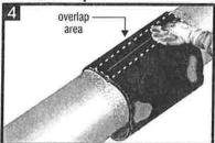
Clean the overlap area of the sleeve with a dry rag where the closure seal is to be applied.
