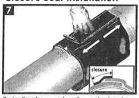
Centre the closure seal on the overlapping sleeve. Using a gloved hand, press from the centre to the ends to ensure good contact is made between the entire closure seal and sleeve. Ensure the entire closure area has been firmly pressed down.
