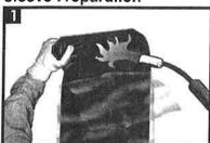
Partially remove the release liner from the sleeve and gently heat the underlap approximately 150 mm (6") from the edge.
